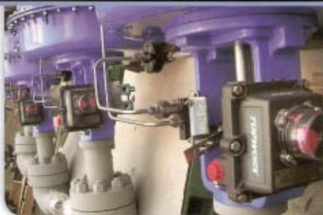
Valvetop D-Series on linear globe valves
